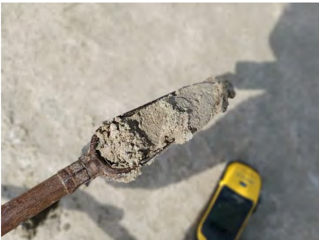
Picture 47: RW007JLM Bearing: N/A Date: 5/17/2021
