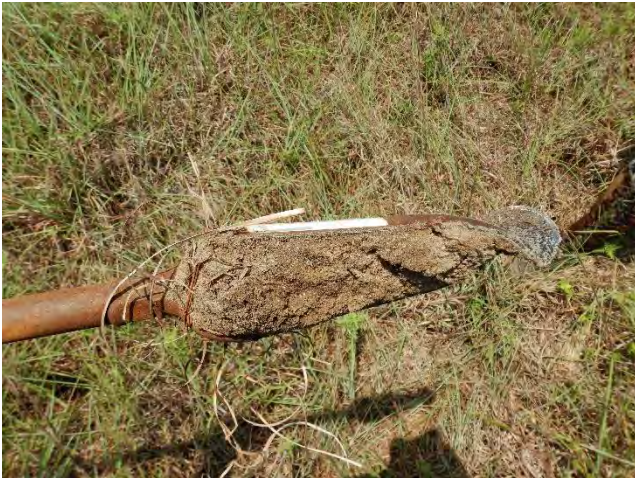
Picture 3: RU001BPH Bearing: South Date: 5/17/2021
