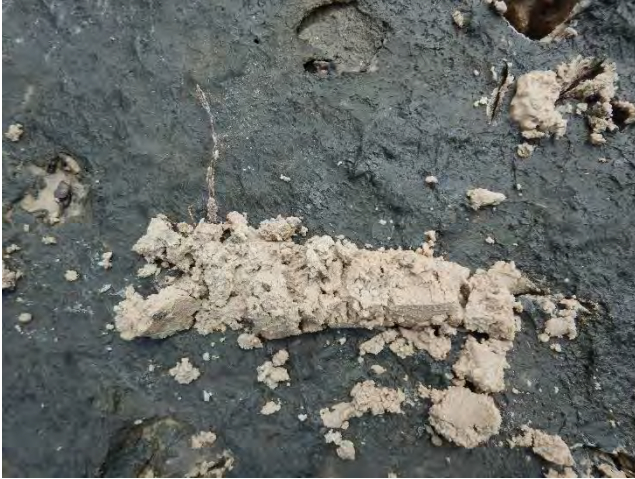
Picture 37: RW006BPH Bearing: N/A Date: 5/17/2021
