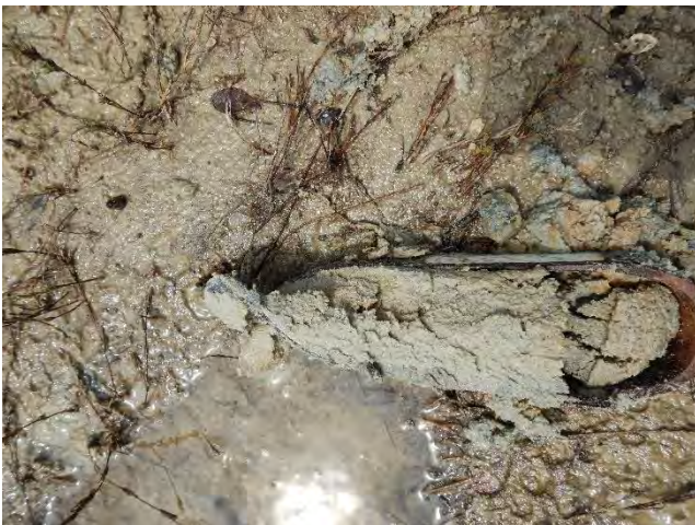
Picture 29: RW005BPH Bearing: N/A Date: 5/17/2021
